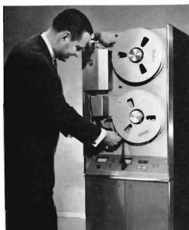
FIG. 2. Second step in operation of TR-3 Player: THREAD THE TAPE.
