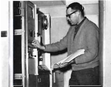
Leonard Gostin, station engineer, checks TR-4.
