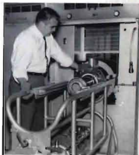
Klystron change is accomplished in only a few minutes with this unique carriage.
