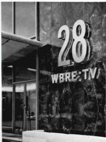
FIG. 3. Entrance to new office and studio building of WBRE-TV, Channel 28, Wilkes-Barre, Pa.
