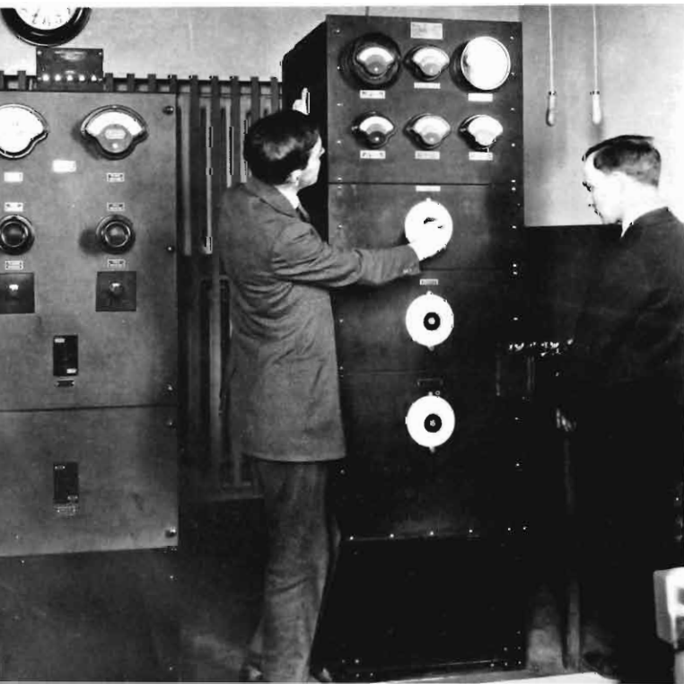
WTIC, 1925. Shown here is the first transmitter installed at WTIC. Mr. Taylor is at the right. The Western Electric 500-watt transmitter will be recognized by many old-timers since it was the transmitter used by a large number of the broadcast stations on the air in the mid-twenties.
